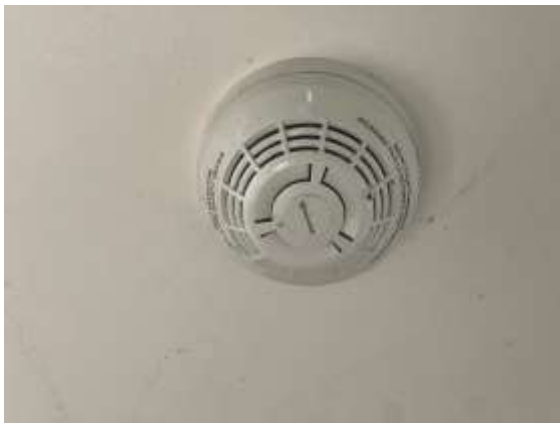
Rate of Rise Heat Detector
